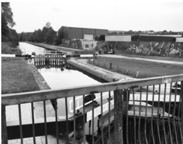
Image above: Sheffield to Keadby Canal, Templeborough
